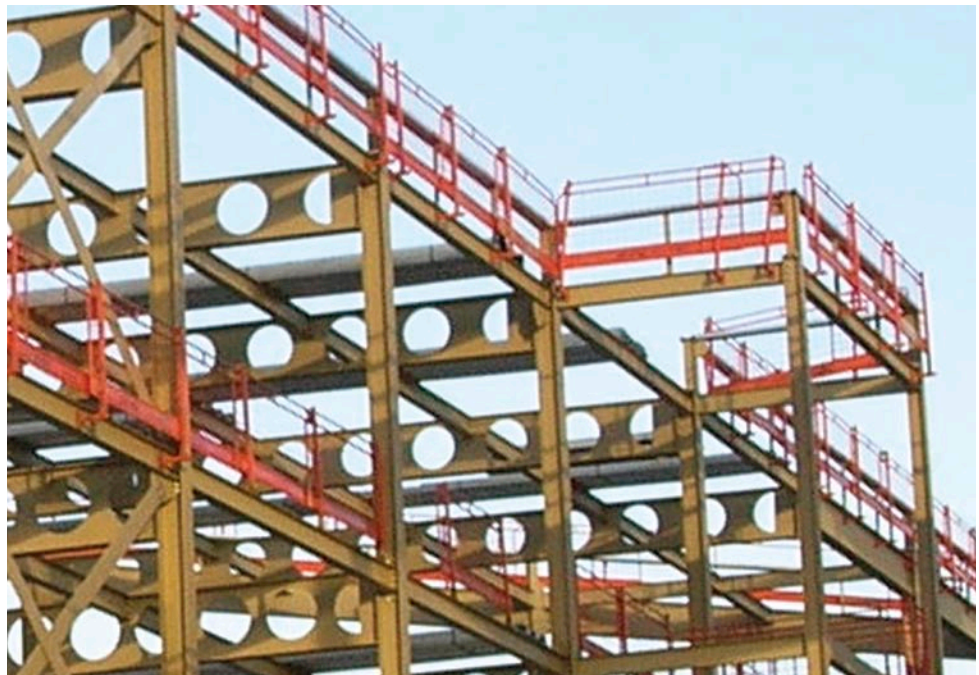
Figure 28 Edge protection installed with the steelwork
