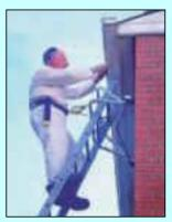
Microlite and ladder belt restraint in use
