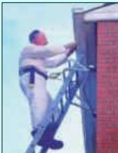
**Microlite and ladder belt restraint in use**
